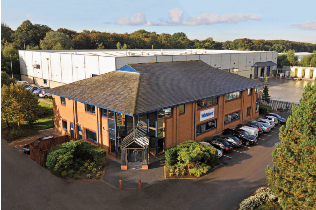
Whitford's new home at 11 Stuart Road, Manor Park, Runcorn
